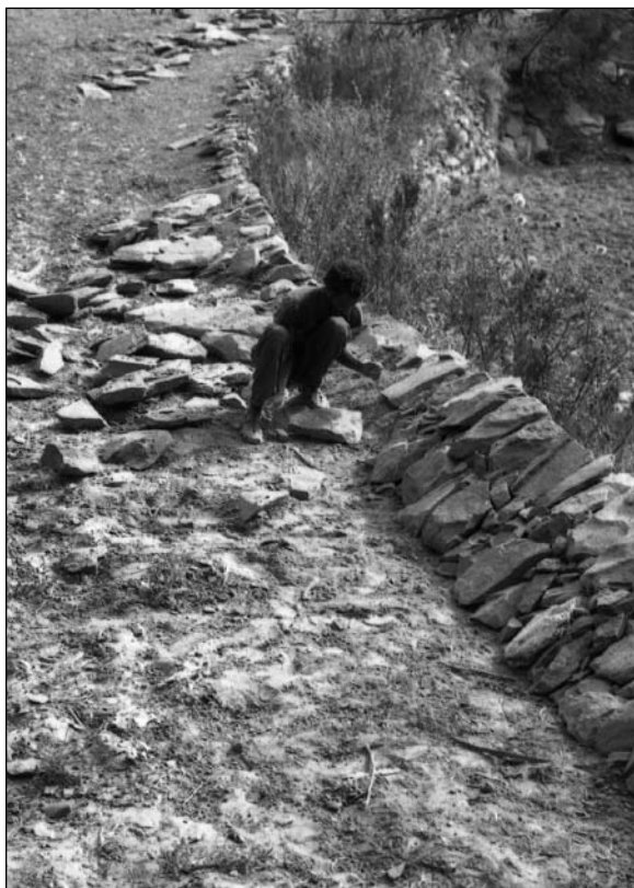
Local initiative in managing soil, stones and water to create land for crop production in Irob District of Eastern Tigray
