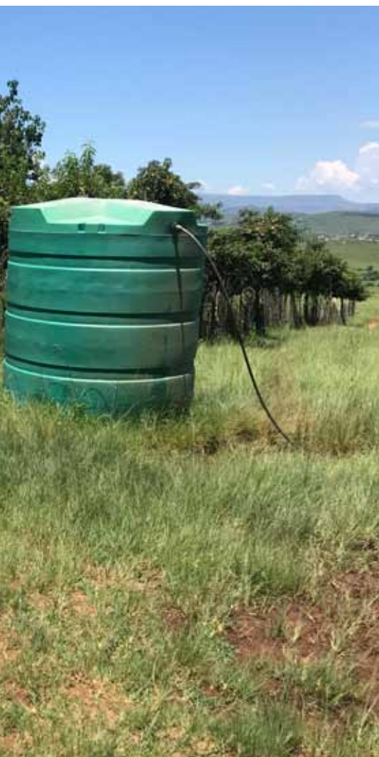
improves the pressure of the water to the households.
