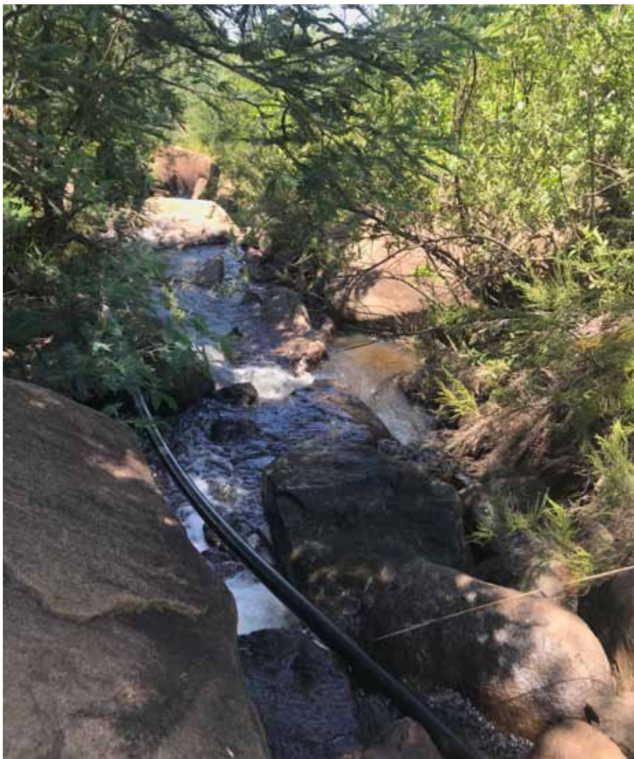
The pipe in the stream in the mountain that supplies households at Mapanekeni.
